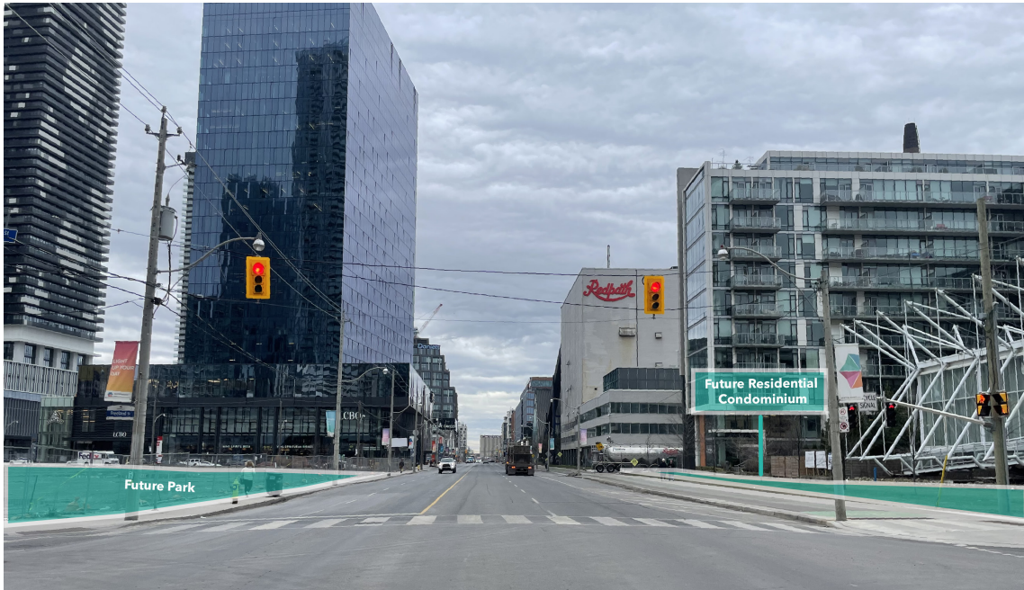
AREA OF QUEENS QUAY EAST WITH MINIMAL STREET-FRONT RETAIL AND ACTIVATION
